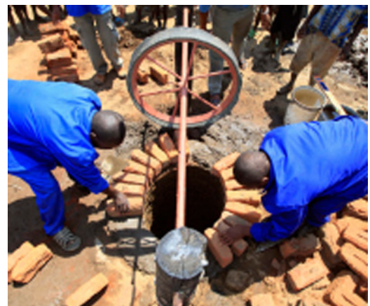
Example of the fair water provision FWC seeks to support e.g. new PumpAid Elephant Pump in Maumsiyeko, Malawi
